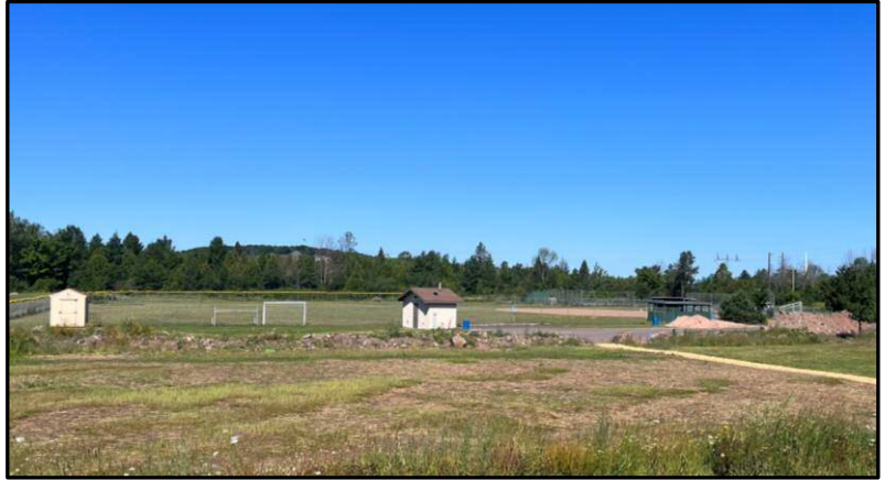
Hurontown Recreation Area Bathrooms & Ballfield
