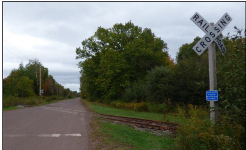
This inactive railroad crossing near the Industrial Park is set to be removed in a 2020 road project.
