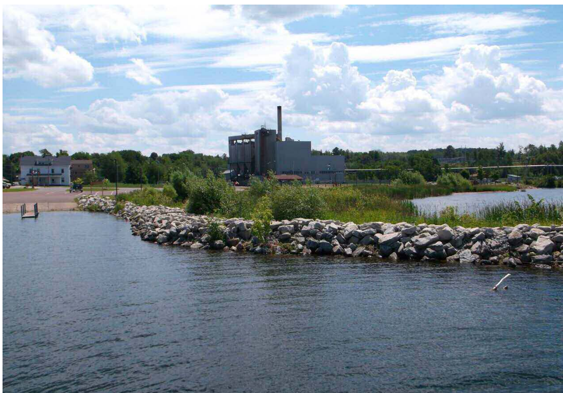
Photo 8: South pier near shoreline & boat launch Note: Sedimentation on south side and vegetation growth
