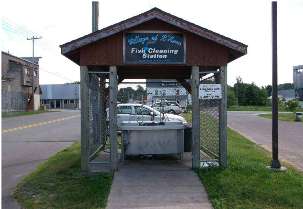
Photo 15: Fish Cleaning Station adjacent to Boat Launch
