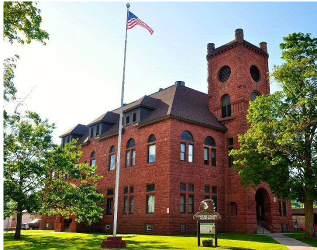
Gogebic County Courthouse, Bessemer, MI (Photo: Skye Marthaler)
