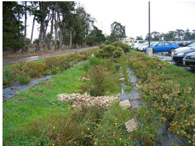
Bioswales are vegetated, mulched, or xeriscaped channels that provide treatment and retention as they move stormwater from one place to another. Vegetated swales slow, infiltrate, and filter stormwater flows. As linear features, they are particularly well suited to being placed along streets and parking lots.
