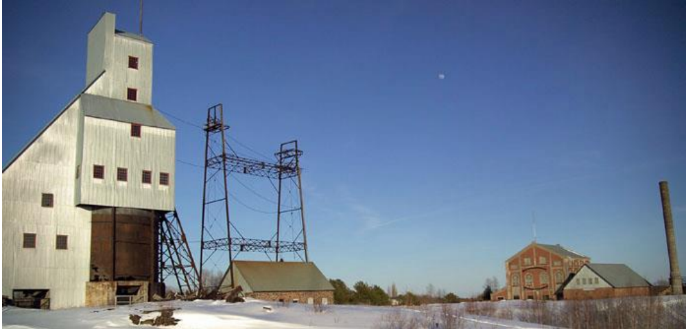
The Quincy Mine #2 Shafthouse (left) and the Hoist House (right). The steam hoist, still located inside, is the largest steam hoist in the world. (Photo: Keweenaw National Historical Park, Dan Johnson)
