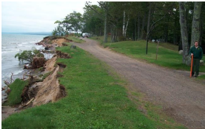
Shoreline erosion at McLain State Park, 2016 (Photo: Michigan DNR)
