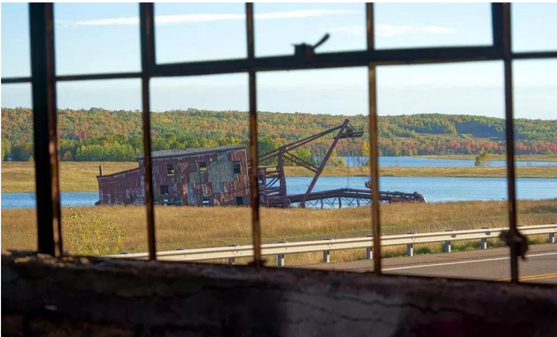
Pictured above is the Quincy Dredge #2, located in Torch Lake just south of Hubbell and across the street from the stamp mill. Photograph by Daniel Woodrum, May 2018
