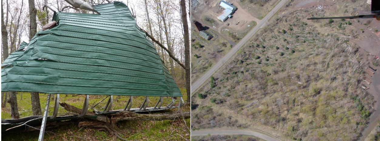
Surveyed tornado damage following an April 30, 2010 event (Source: NWS Marquette).
