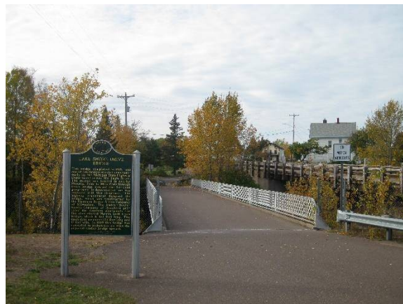
Eagle River Bridge (Source: Richie Diesterheft)
